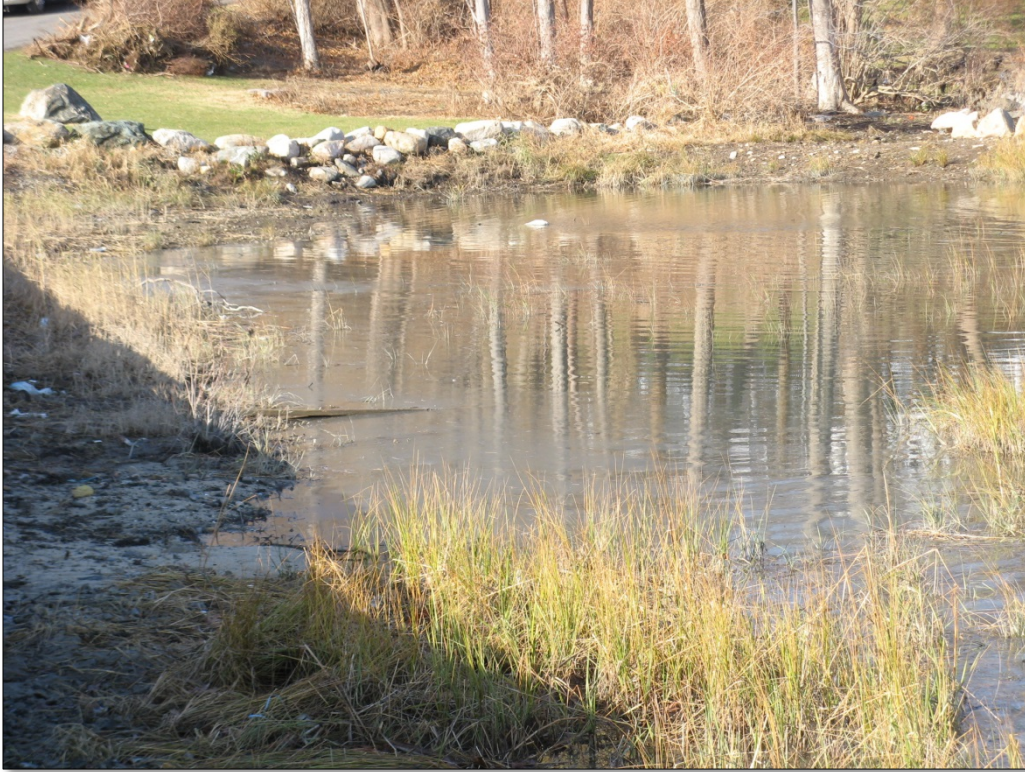
Photo 3 - Post Restoration, Facing West on November 28, 2012.
